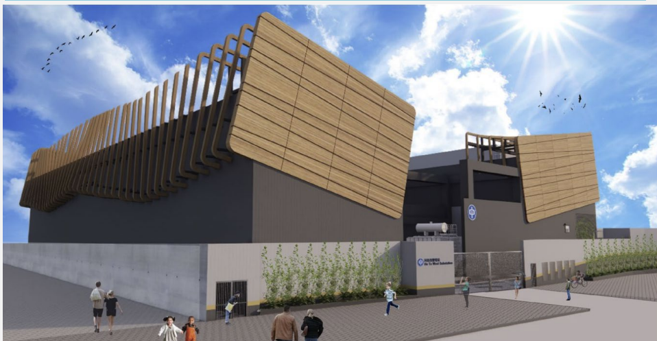
Ho To West Substation
