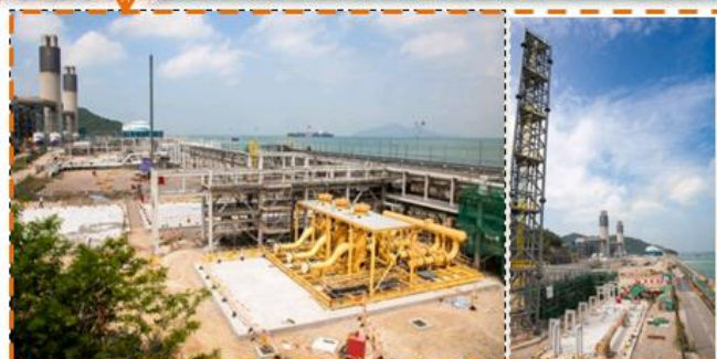
A new gas receiving station is being built for WEPII gas
